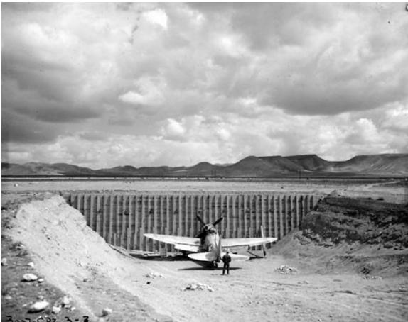
Positioning F-47 in 16 foot revetment at 4000 feet from GZ
